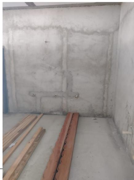
INSTALAÇÕES HIDROSSANITÁRIAS – ENCANAMENTOS, CONEXÕES E REGISTROS NOS SANITÁRIOS. RASGOS NAS PAREDES JÁ COBERTO COM CHAPISCO E REBOCO.
