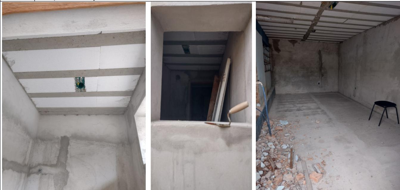
INSTALAÇÕES ELÉTRICAS – CONDUÍTES E CAIXAS DE PASSAGEM. RASGOS NAS PAREDES JÁ COBERTO COM CHAPISCO E REBOCO.
